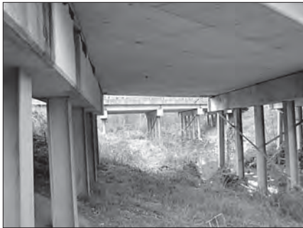
Sunny Meade Creek Trail corridor at Interstate 540
