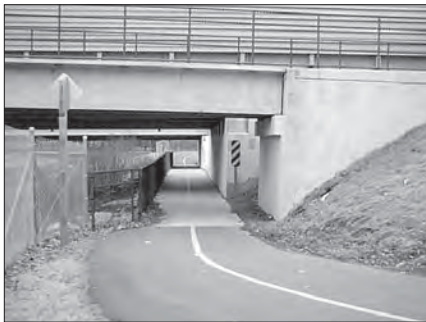
Trail Underpass with Railing
