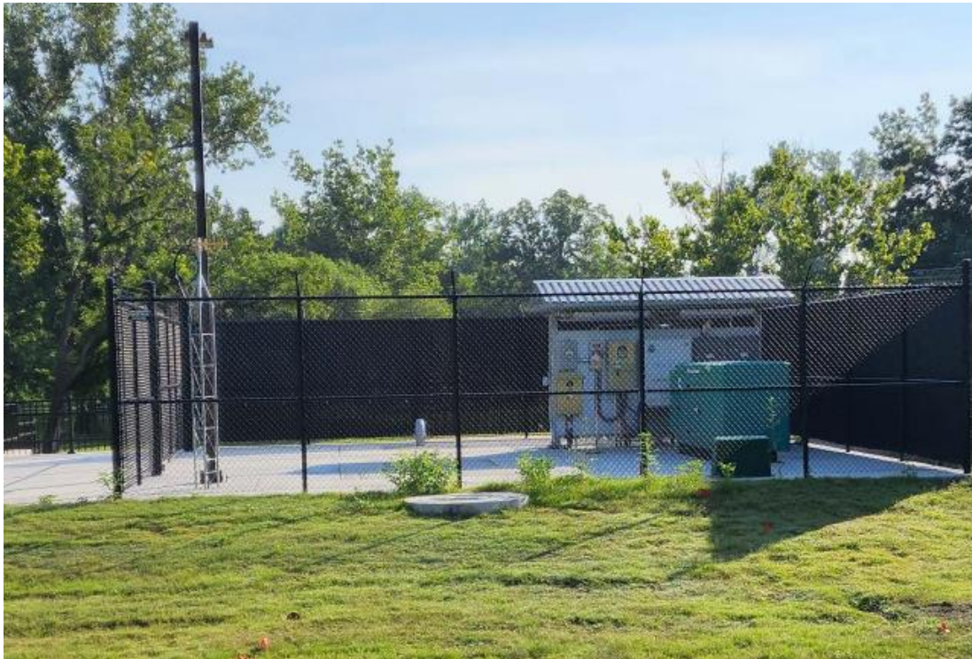
Pump Station 28: Photo taken July 24, 2023
