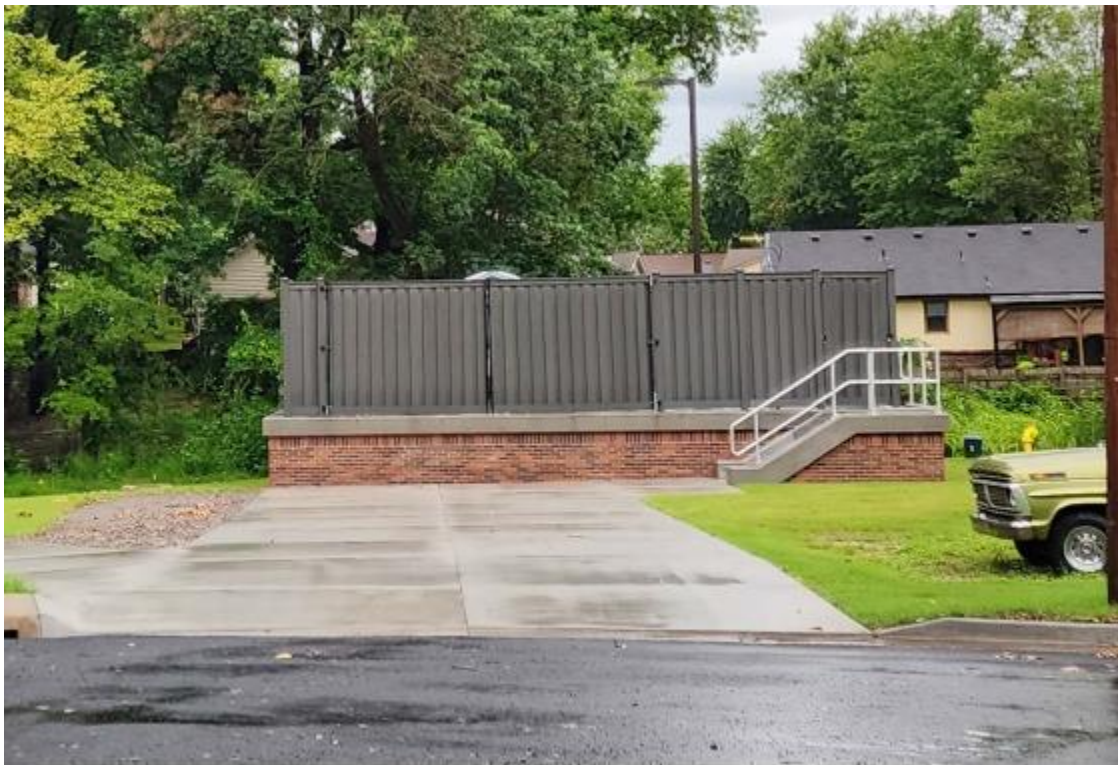
Pump Station 29: Photo taken July 21, 2023
