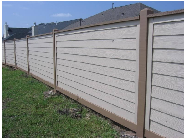
6 ft Hardiplank Fence, 6×6 Exposed Posts With Cap and Trim
