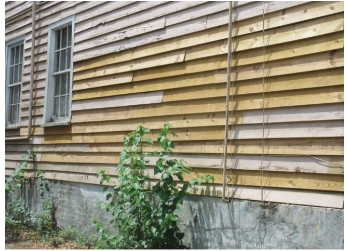
Figure 3: Incremental repair is best done using in-kind material to minimize differences in the performance characteristics that could negatively affect the overall assembly. Photo: NPS.
