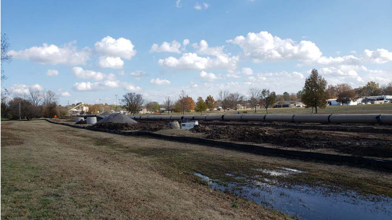
Preparation For Laying Pipe Across MLK Park
