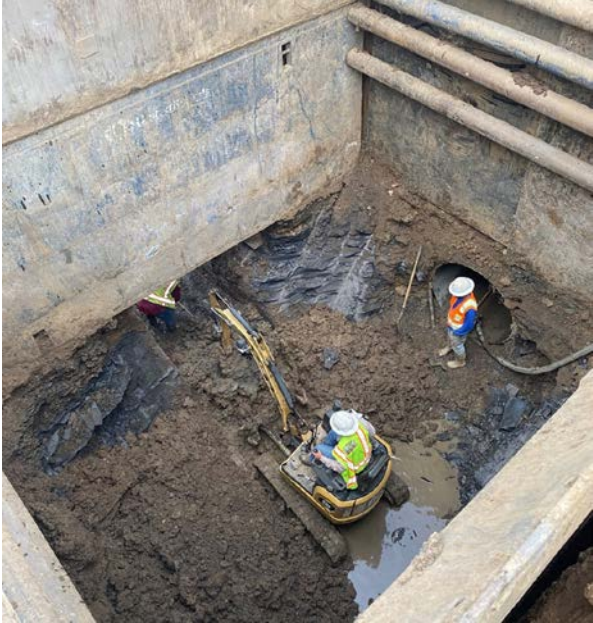
Mini Excavator Clearing Spoils From Tunneling Under Greenwood Avenue
