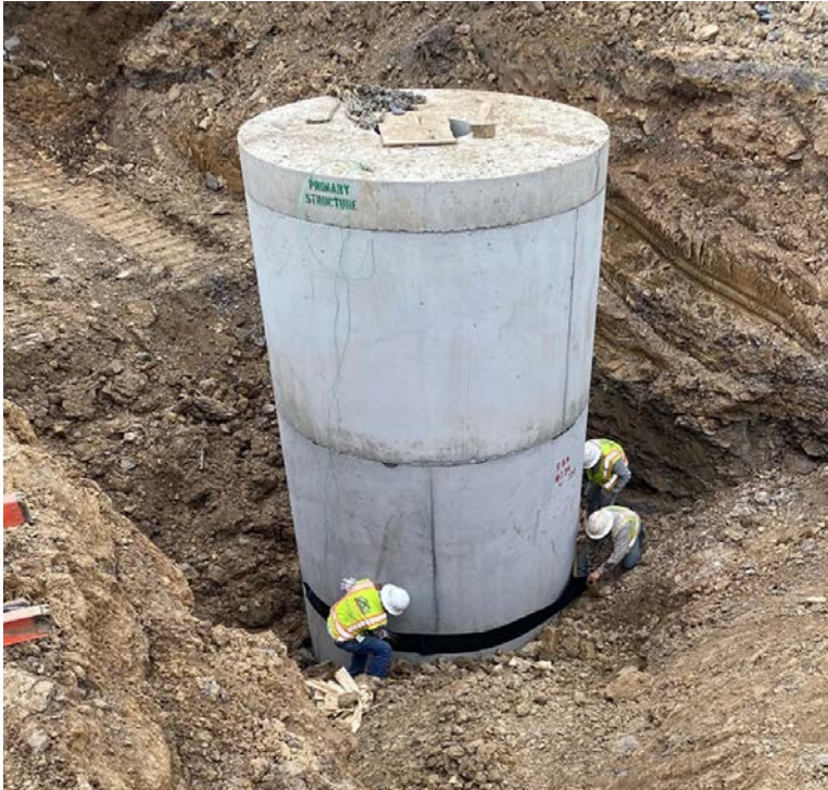
Setting Precast Manhole
