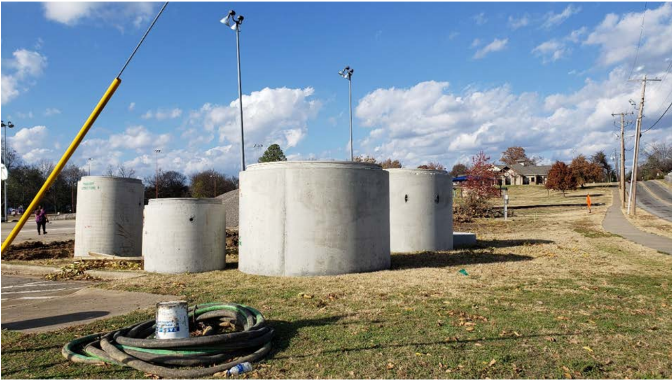
Stockpiling Precast Manholes
