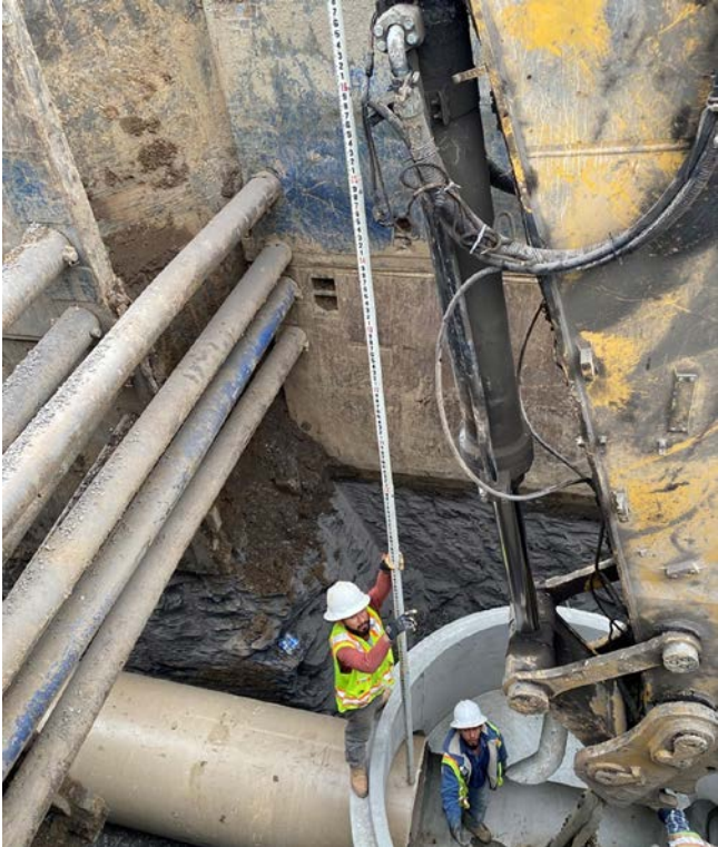
Connecting 42-Inch Diameter Pipe To Manhole
