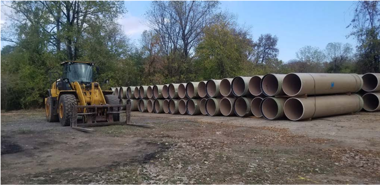
Stockpiling 42" Fiberglass Pipe
