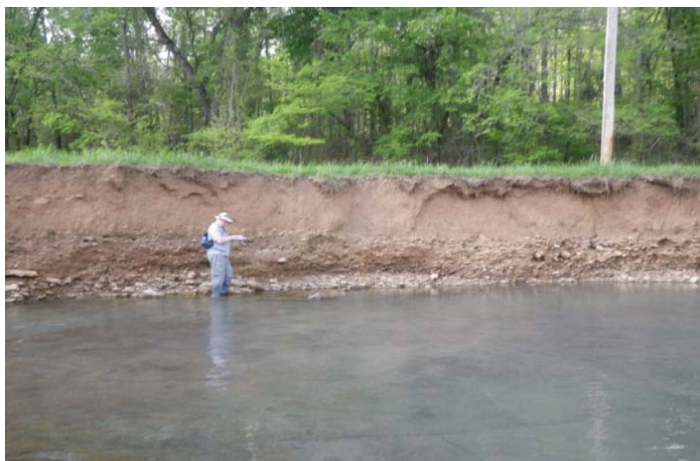
Figure 17. Stream bank with very high bank erosion hazard in the Upper Frog Bayou watershed.
