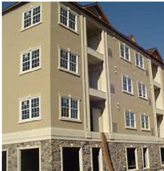
Image showing a building with accent materials (stone and stucco with banding highlights)
