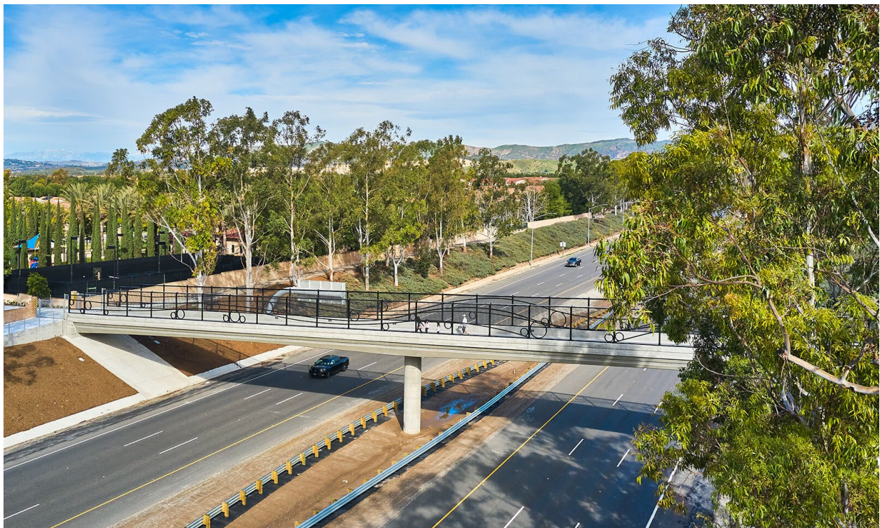
Figure 8. This pedestrian bridge in Irvine, CA offers safe passage over a highway for pedestrians. The bridge serves as a vital link to the city’s trail network. Successfully linking the west parcel and the east parcel of the ACME Brick will be vital.
