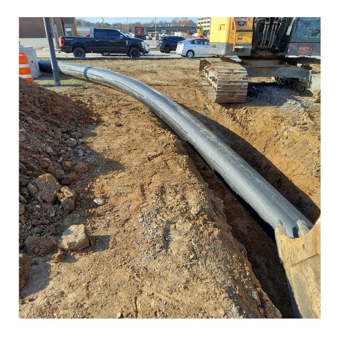
Horizontal Directional Drilling – 18-Inch Pipe Being Pulled Into Bore Hole
