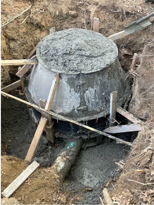
Formed In Place Manhole
