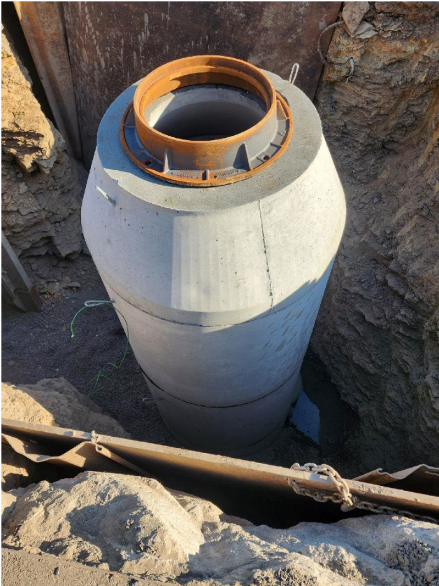
Line 8 – Manhole Installation In Rock
