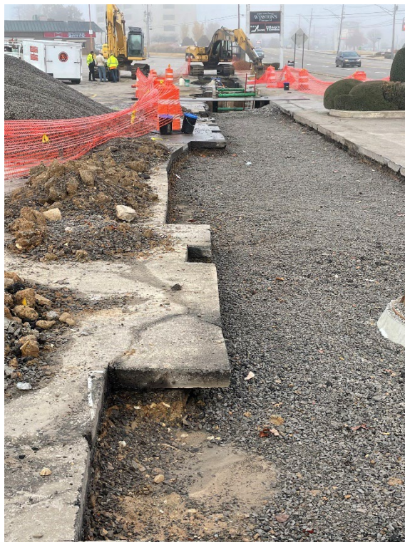
Line 8 - Prepping Sub-Base For Asphalt Patch
