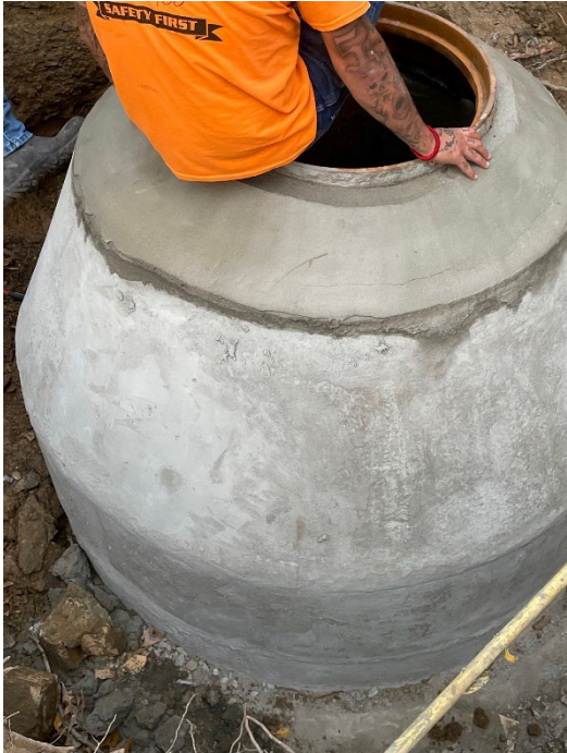
Finishing Formed In Place Manhole
