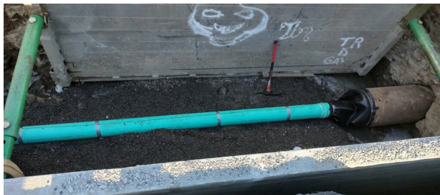
Pipe Under Box Culvert Casing End Seal
