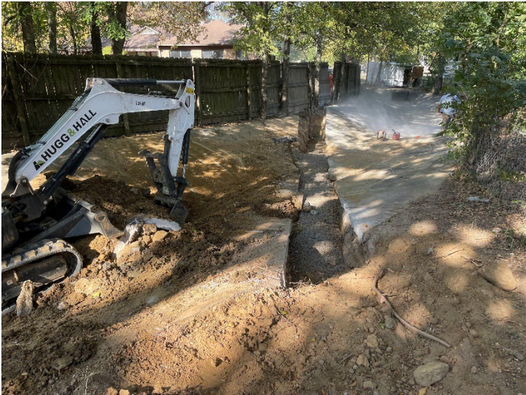
Line 4 – Concrete Lined Storm Drain Cut For Pipe Installation
