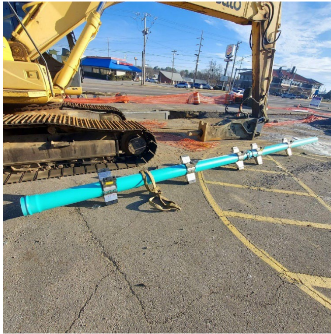
Line 8 – Pipe With Spacers For Insertion Into Casing Under Box Culvert
