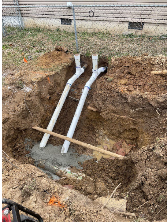
Lateral Service Lines and Clean Outs
