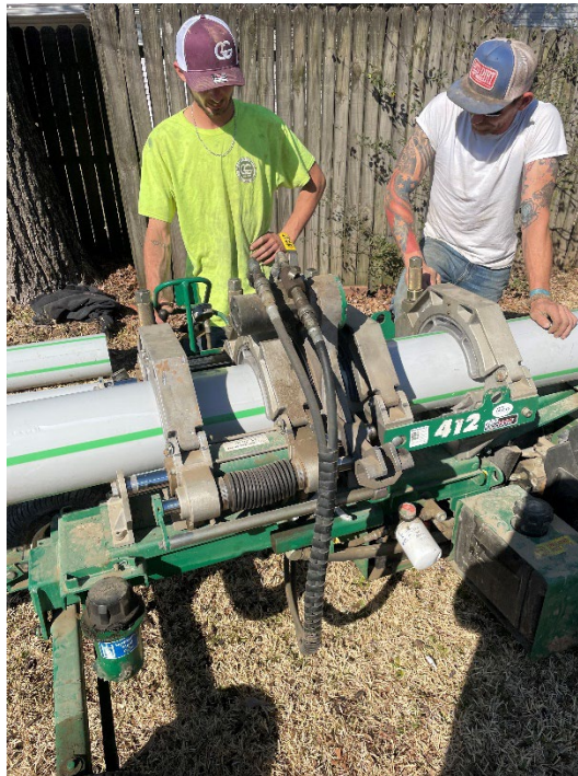
Fusing HDPE Pipe
