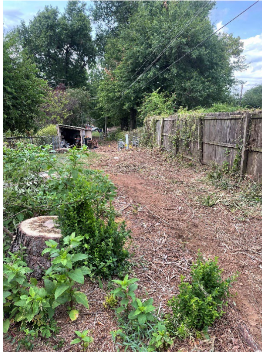
Clearing and Grubbing
