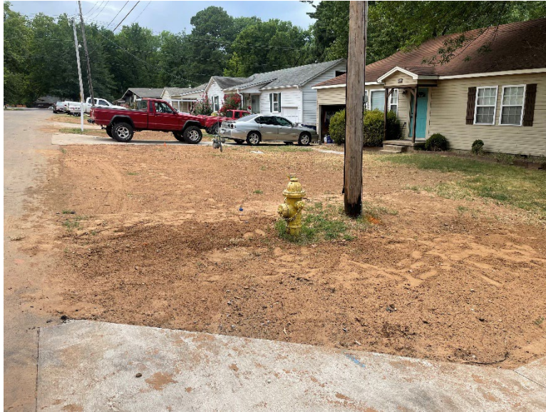
Preparing Surface Restoration
