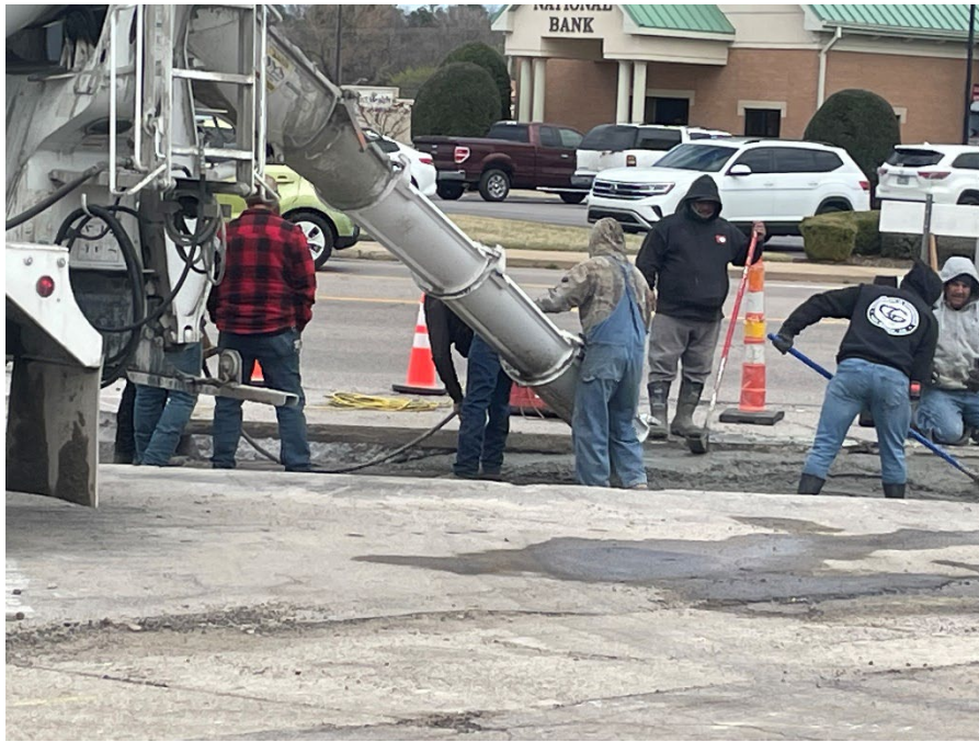
Line 8 – Placing Base For Asphalt Patch
