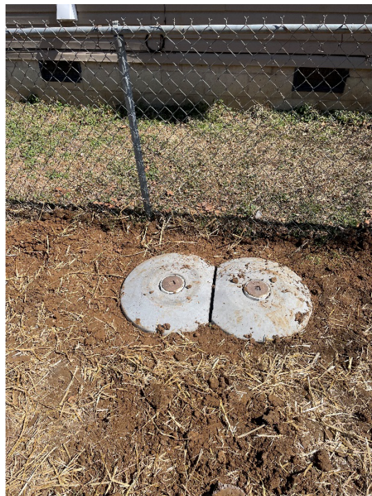
Finished Clean Outs
