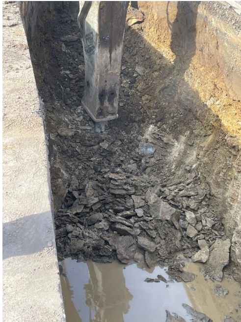
Line 8 – Rock Excavation
