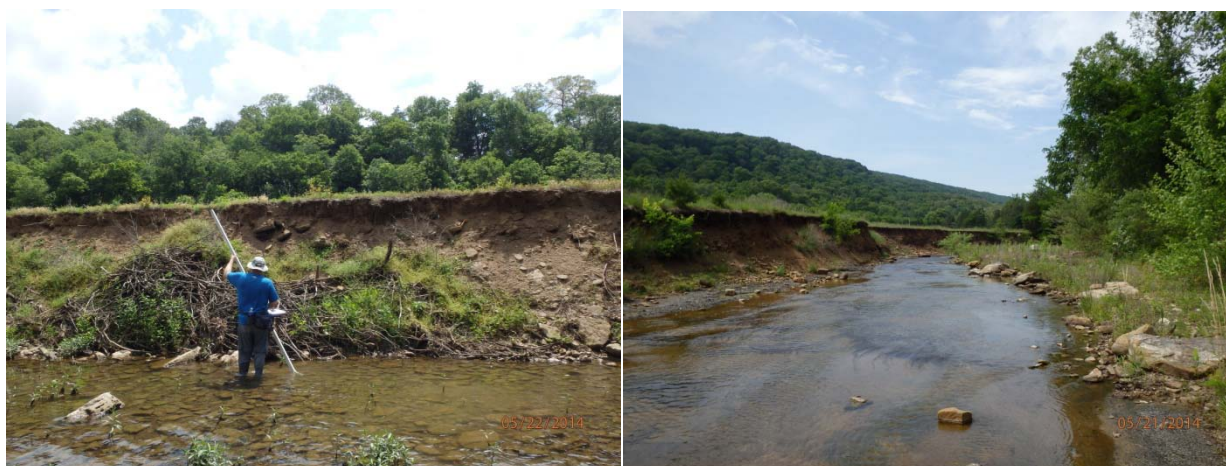
Figure 35. Streambank erosion on CC and the MFC.
