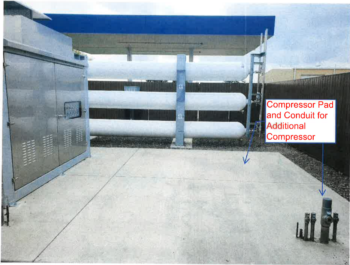
Storage Vessel Pad and Tubing for Additional Storage and Slow Fill Connection
