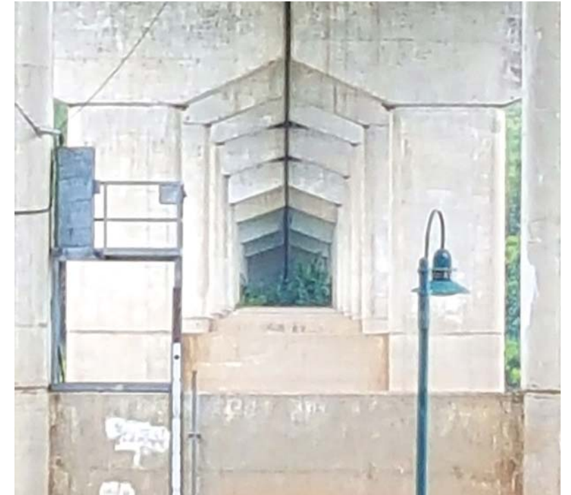
U.S. Highway 64 Bridge (Source: Gateway Planning)
