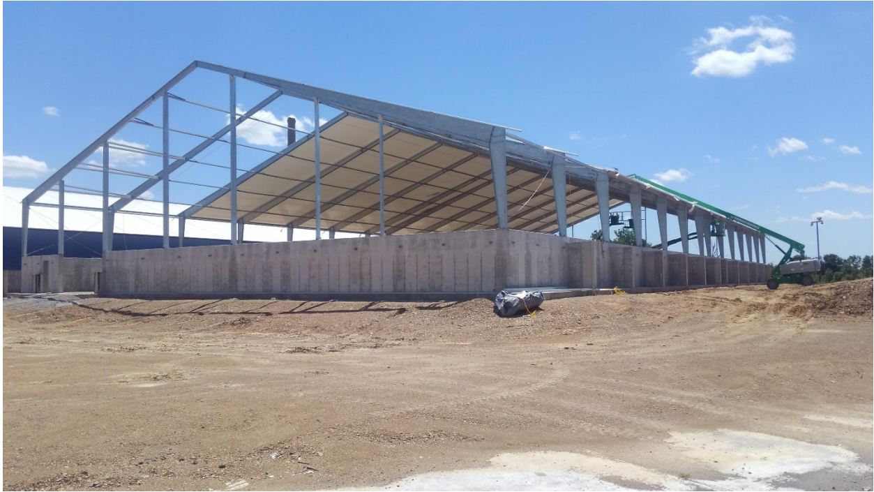
Framing for Warehouse 2 nearing completion.
