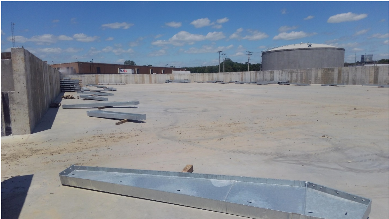
Steel framing for Warehouse 1 placed and ready to begin installation.
