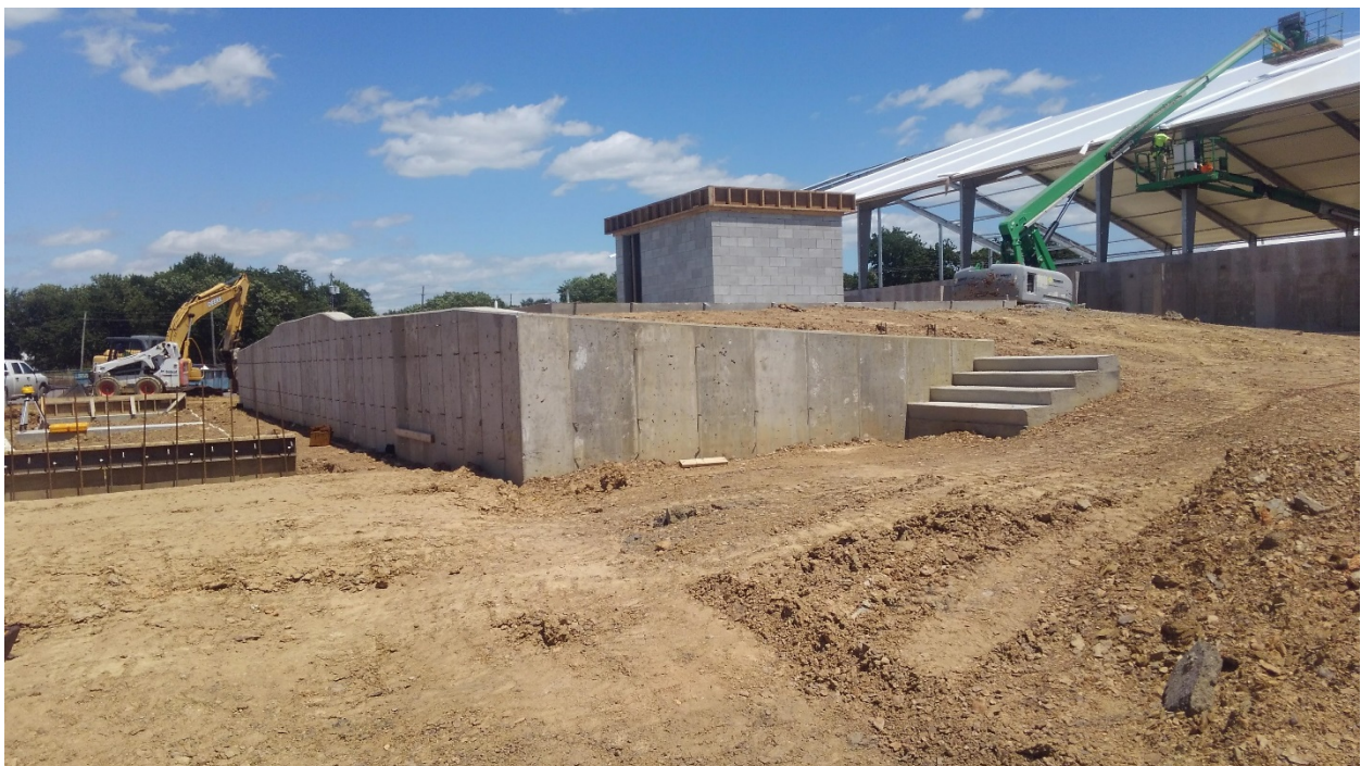
Concrete retaining wall and steps completed at Office / Scale House.
