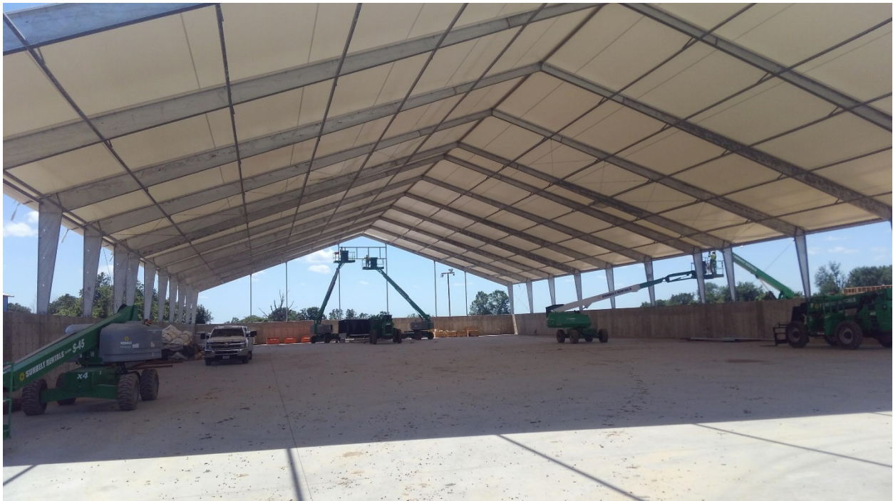
Roof covering for Warehouse 2 80% complete.
