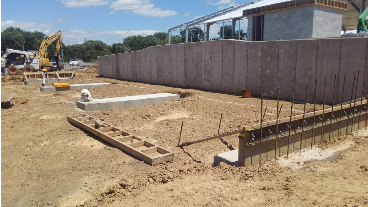
Foundations poured for Truck Scale.
