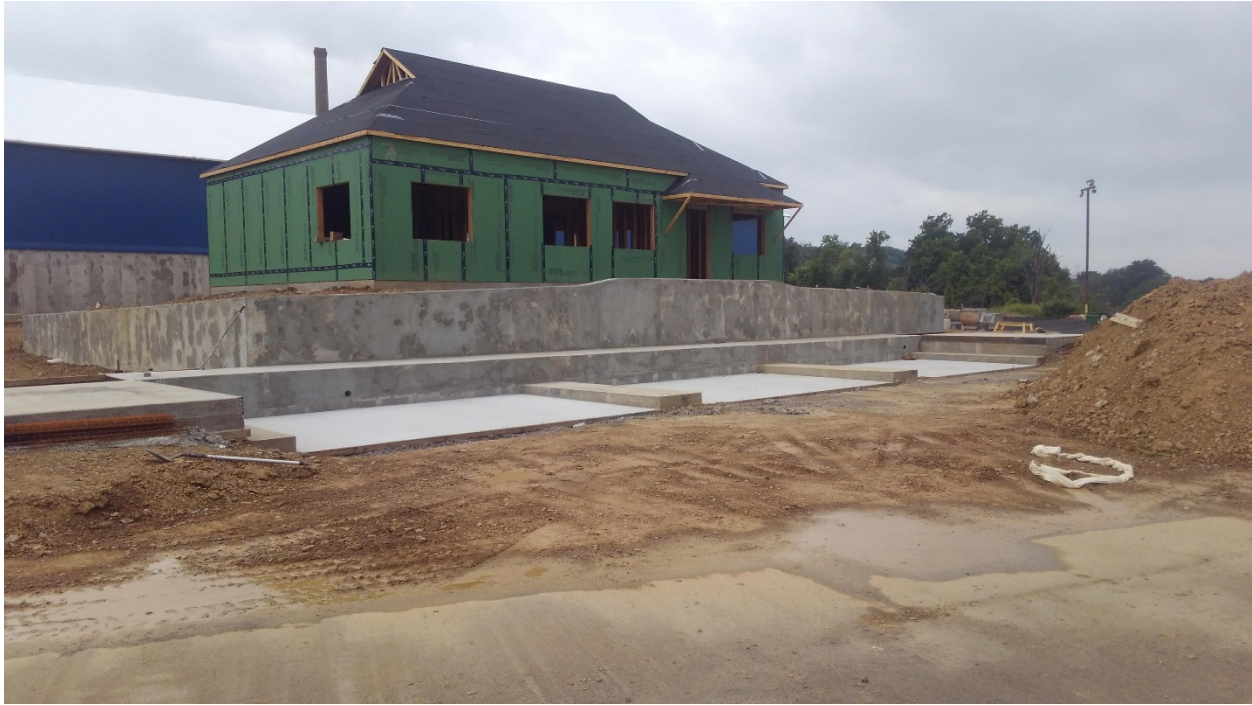
Scale House / Office – North Side. Building is framed and sheathed.
