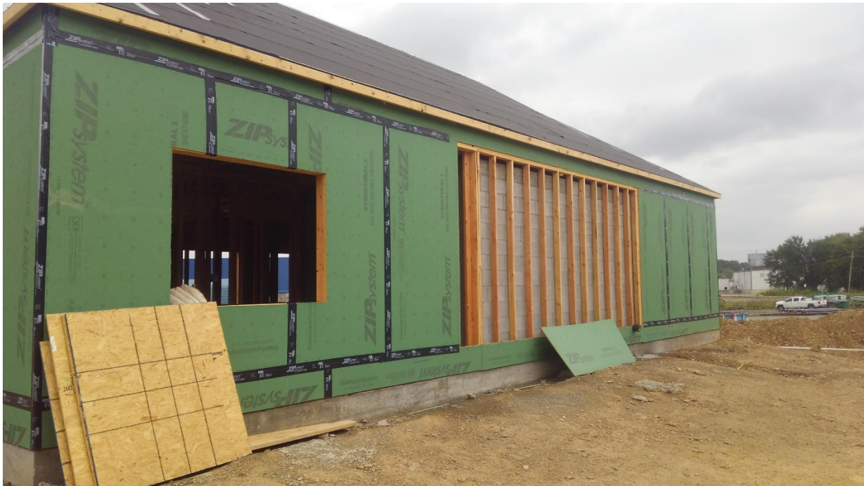
Scale House / Office – West Side. Building is framed and sheathed.
