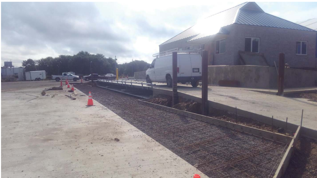
Truck Scale installation is nearing completion with pipe bollards installed.
