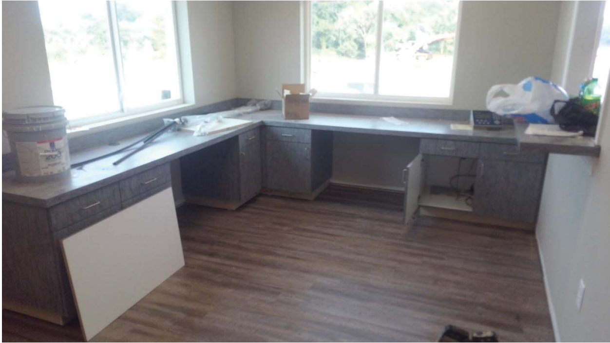
Millwork installation at Scale Office in Scale House / Office.
