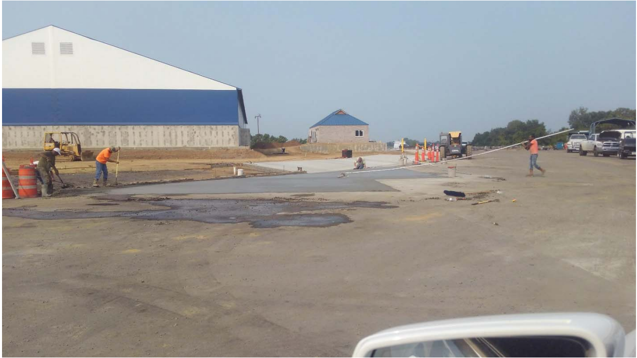
Pavement / drainage swale being finished on the East side of Warehouse 2.
