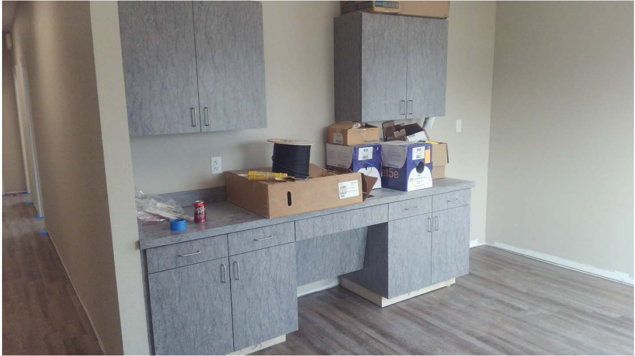
Millwork installation at Break Room in Scale House / Office.
