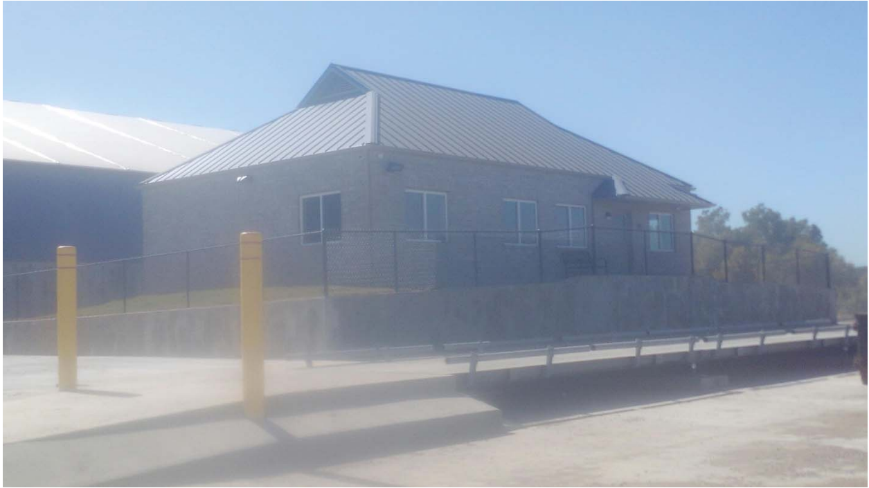
Fencing and sod has been completed at the Scale House / Office.
