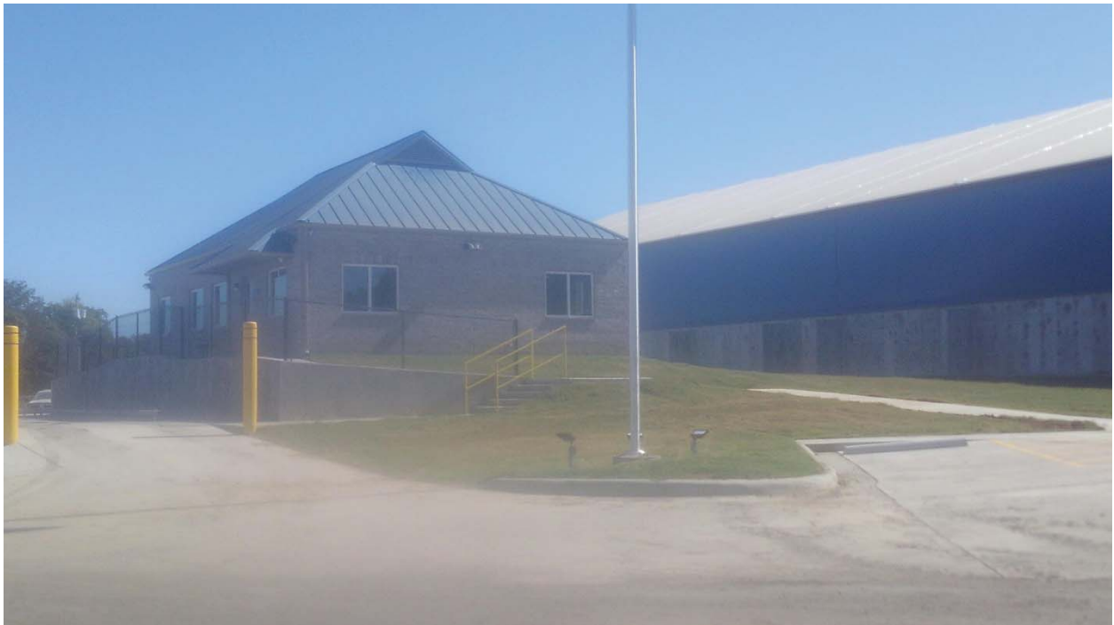
Stair handrails have been completed on the West side of the Scale House / Office.
