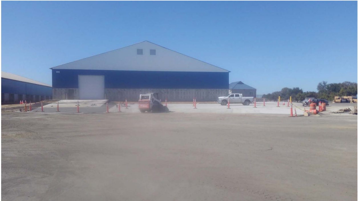
Site pavement completed on the East end of Warehouse 2.
