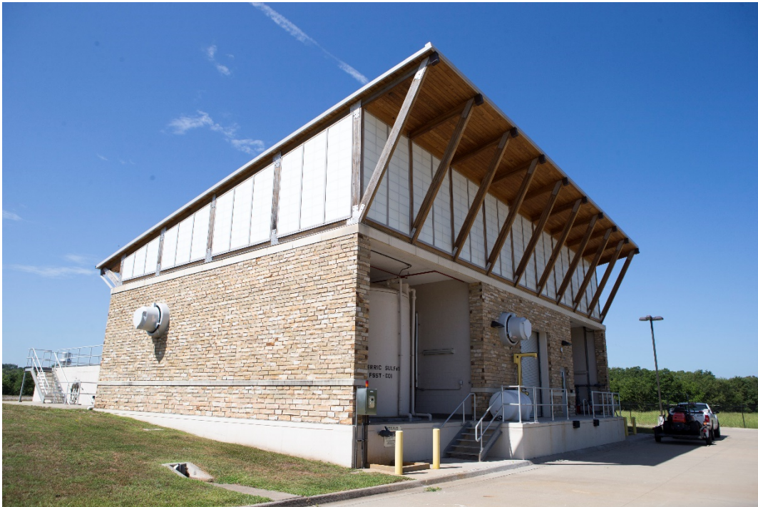
Sunnymede Equalization Basin Chemical Treatment Control Center (pre-2019 Flood)
