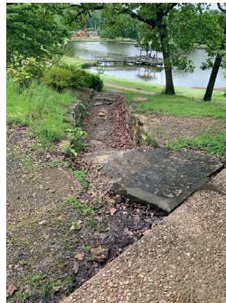
Examples of access points to restrooms and picnic pavilions.
