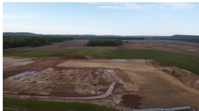
Beginning status of Phase II.
